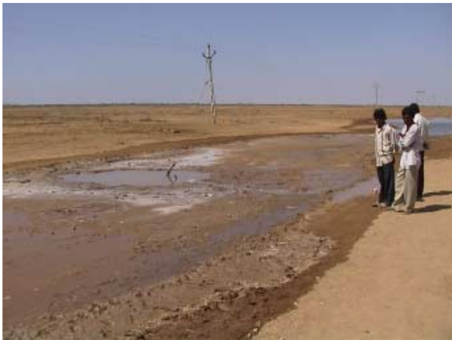
Figure 7. Sand boil and expulsion of salt water to the surface observed near Lodhai at a location to the east of that shown in Figure 6. Water was still oozing out when the authors visited the site on February 23, 2001.
