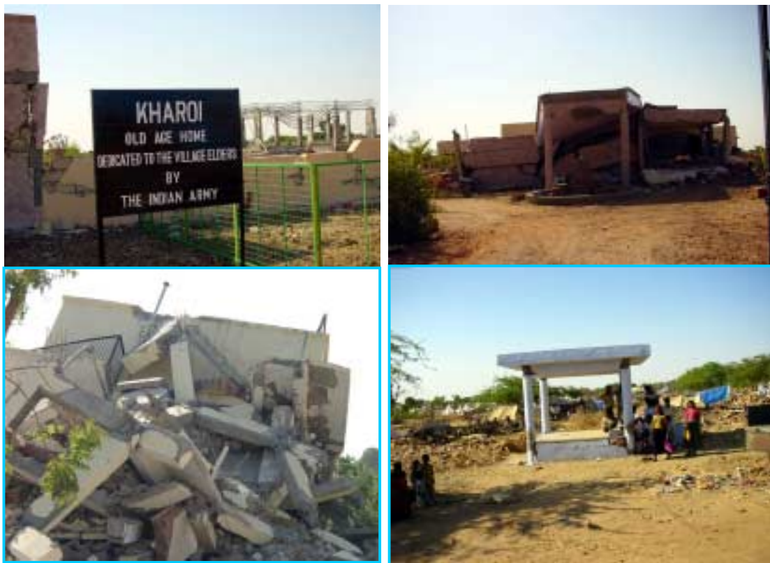
Figure 48. Damage scenes from the Chaubari area, to the east and close to the probable epicentral area. The top two photographs are of the compound of the damaged old age home. Lower left shows the severe nature of damage to reinforced concrete building in Chaubari. The lower right photograph shows the surviving simple concrete structure of a resting place in the midst of a completely destroyed village in Chaubari area, seemingly consisting of non-engineered houses. The tents accommodate survivors can be seen in the background.
