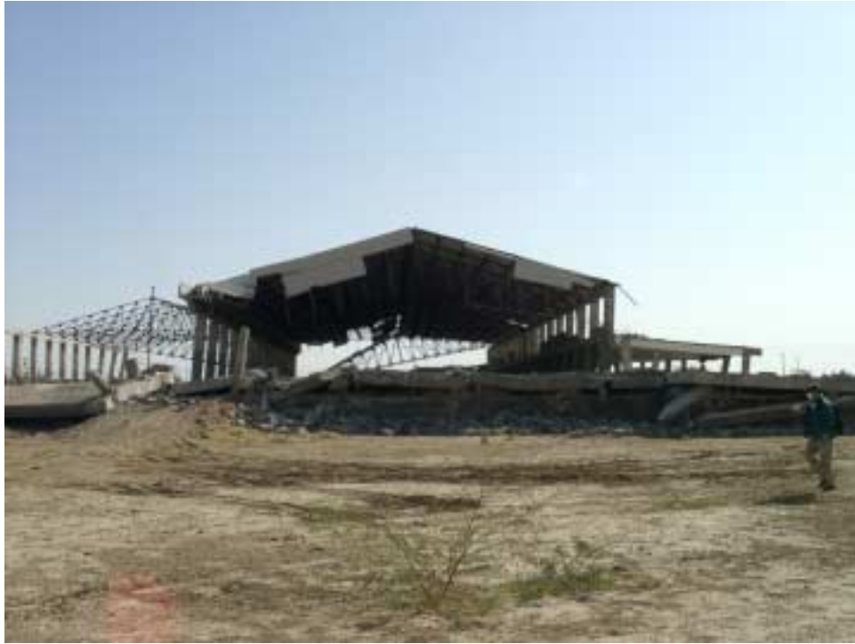
Figure 24. Collapse of the incomplete KC Polytec Ltd. factory building between Dagala and Madhapur, about 20km east of Bhuj. The building had collapsed with large southward movement.
