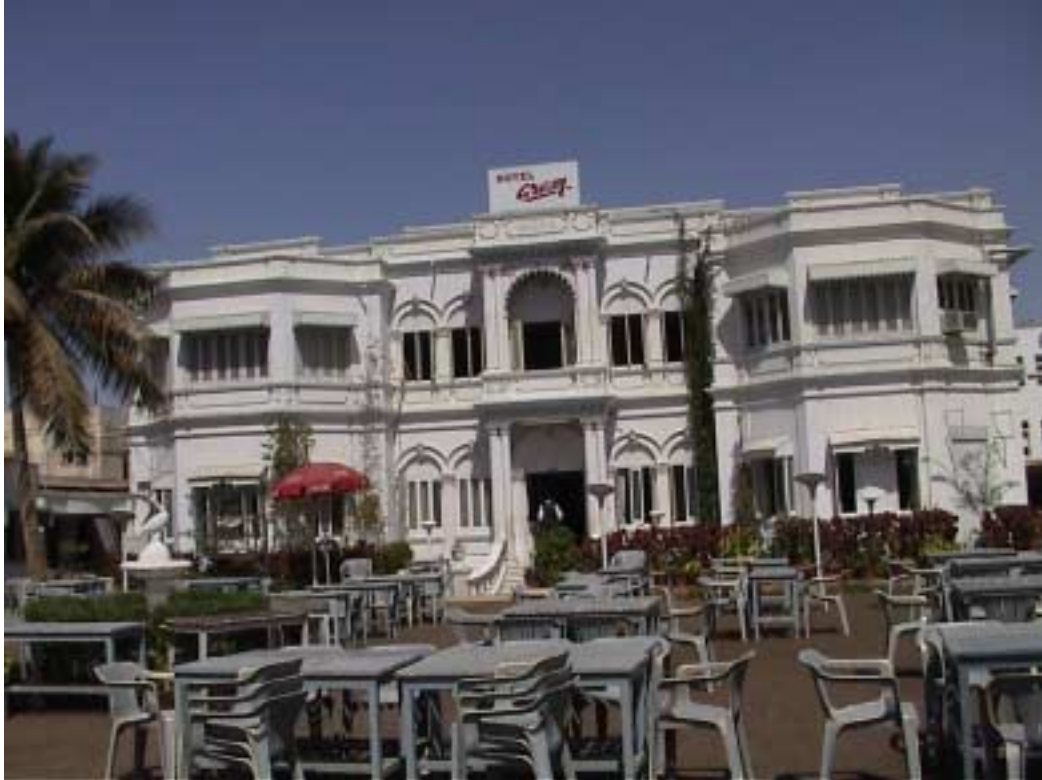
Figure 16. Hotel Aram in Jamnagar, consisting of a stucco building dating back to the times of British India. The building looked intact from distance and it was in business. However, looking closer it was found that the building had many cracks and owner some repair of the damage was undergoing as the hotel was running.
