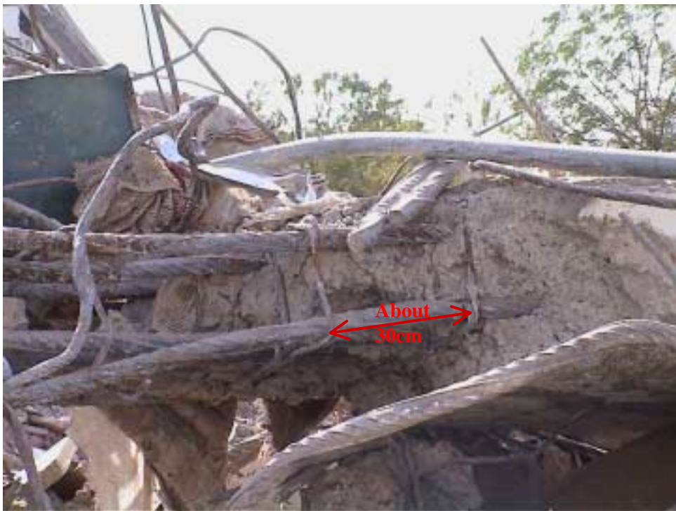
Figure 13. Close-up view of the rubble from Manasi complex, showing the nature of reinforcement placement and the quality of concrete utilized in columns in the collapsed portion.
