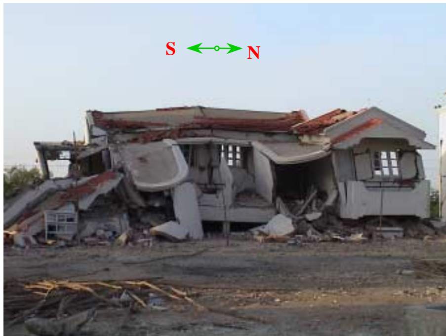
Figure 21. Completely collapsed block of two housing units similar to that shown in Figure 21. It had collapsed completely with large southward movement, which may be due to the presence of stronger north south motion this earthquake.
