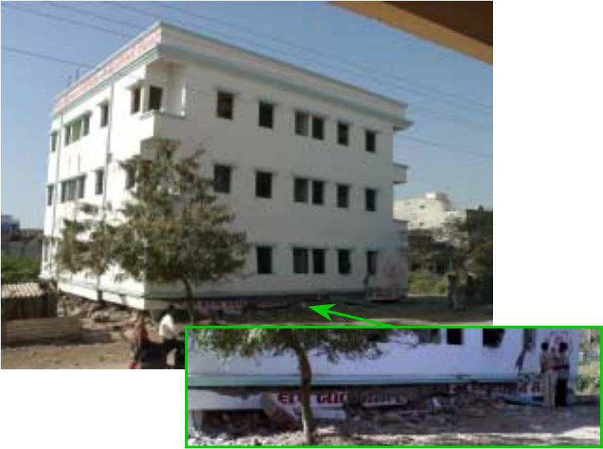
Figure 44. Collapsed ground floor (inset: close-up view) of Children’s Hospital and Research Center in Gandhidham, indicating a typical nature of soft ground floor failure.
