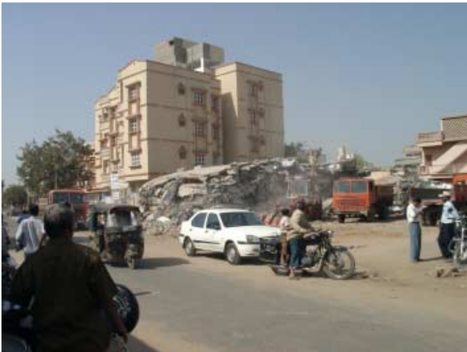
Figure 14. Wreckage of collapsed building and crushed vehicles parked in the open ground floor, near Maninagar station, south east of Ahmedabad. The adjacent building with open first floor parking space sustained some damage mostly due to the impact of collapsed building.
