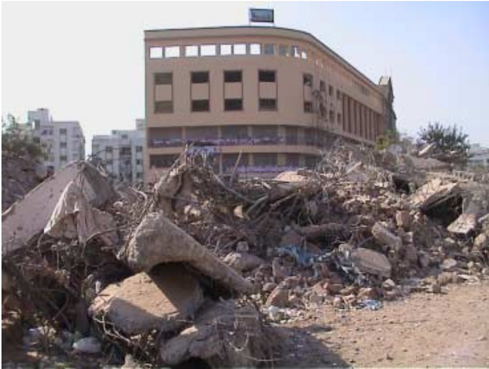
Figure 12. The rubble of concrete and reinforcement from the collapsed portion of the Manasi complex dumped across the street nearby. Most of the buildings seen in the background seem to have little if any structural damage.
