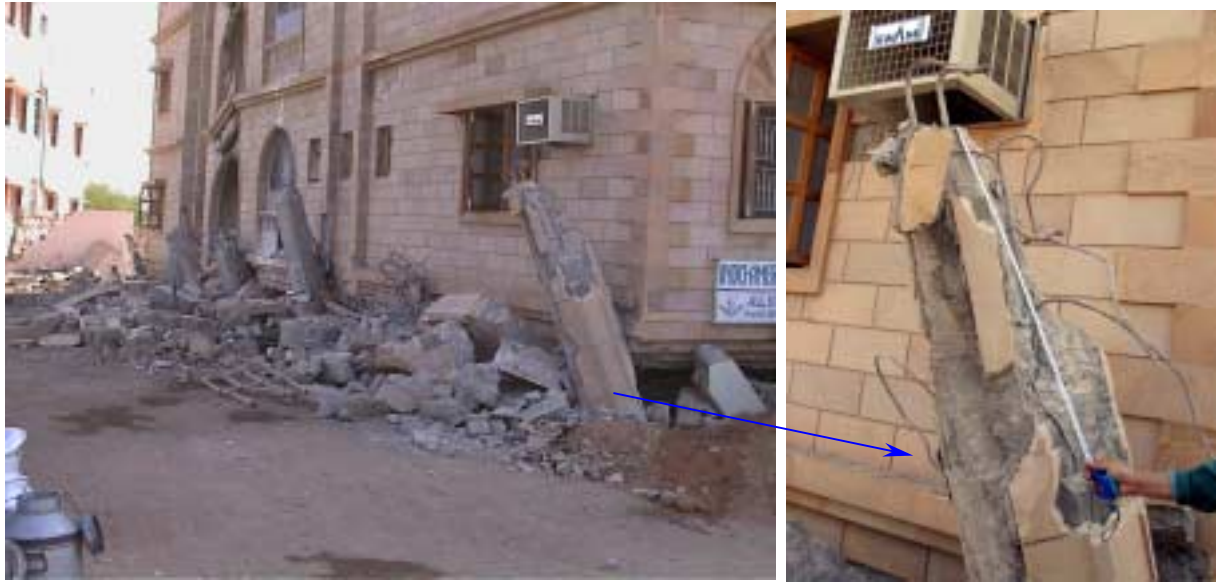
Figure 38. Close-up view of the nature of failure in the ground floor reinforced concrete columns together with a magnified view of column reinforcement with deficient lateral ties for confinement. Also the presence of aggregate in the concrete was difficult to discern.
