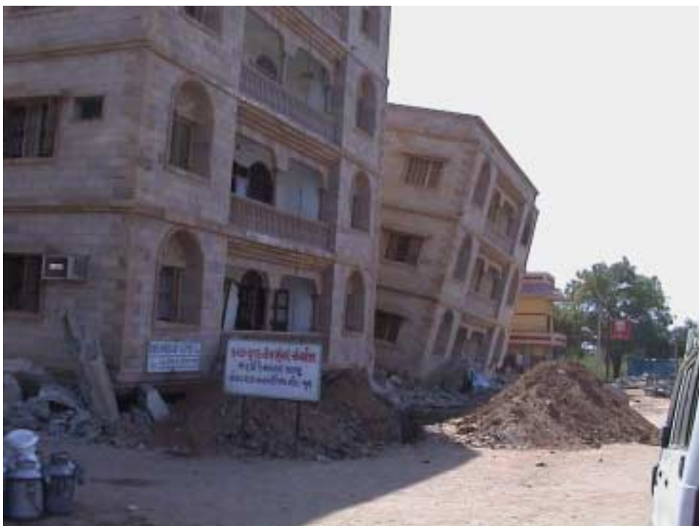
Figure 37. Closer view of collapsed ground floor with store front sign boards sitting on the floor.
