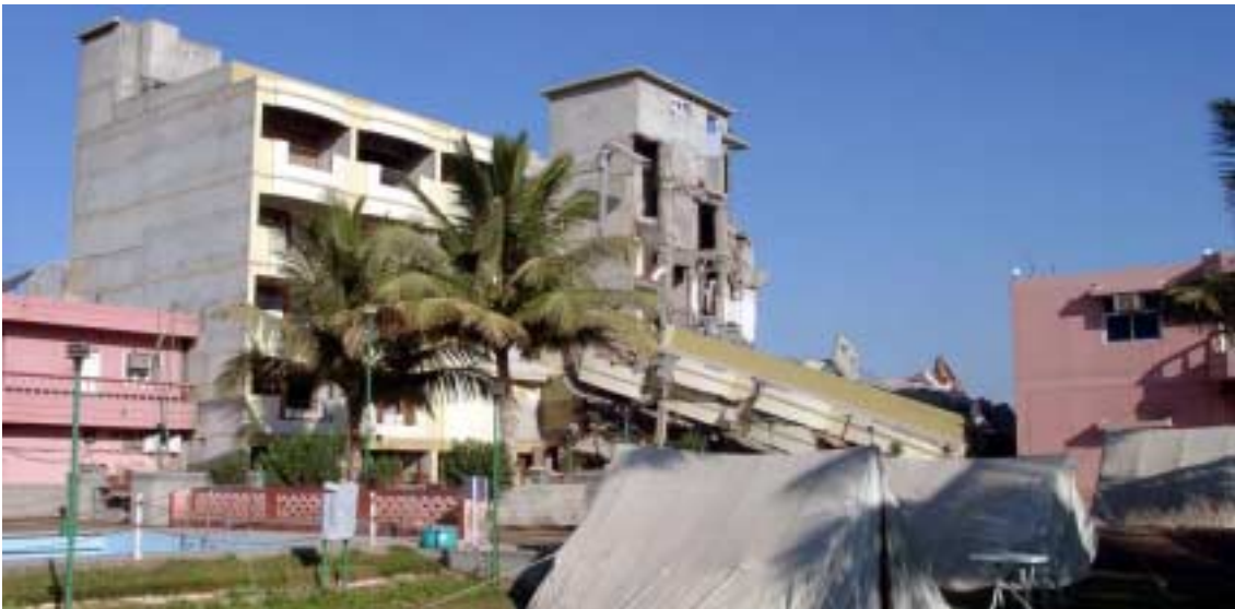
Figure 46. Closer view of the collapsed wing at Sharma Resort. Tents in the foreground were arranged by the owner for renting to the prospective customers. Some of rooms in the blocks that had not collapsed were also available for renting. The authors opted for the tent.
