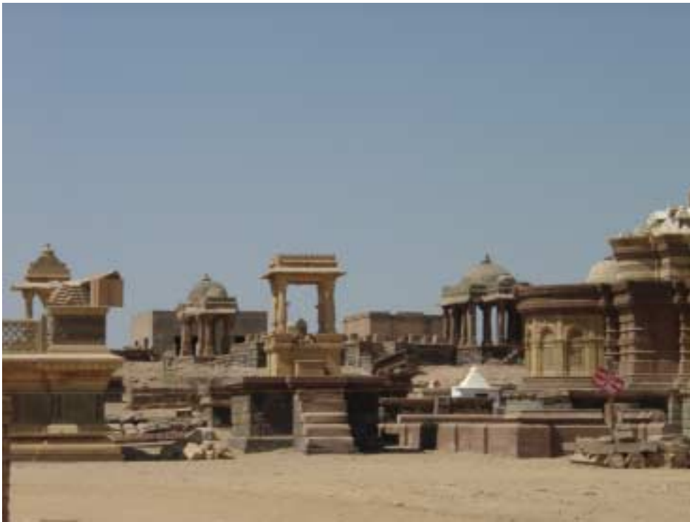
Figure 35. Closer view of the damage to holy burial ground for kings and queens from early days, allegedly from over 200 years ago.
