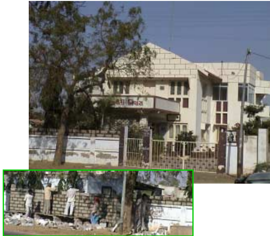
Figure 41. Apparently undamaged residential building adjacent to the community polytechnic, where the repair of the collapsed boundary wall (inset) was in progress to the left of entrance gate.
