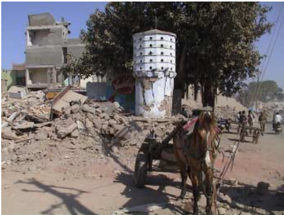
Figure 39. Badly cracked but standing pigeon house in the midst of total devastation of human habitation all around in Anjar. The supporting structure of pigeon house consists of masonry in mud mortar.
