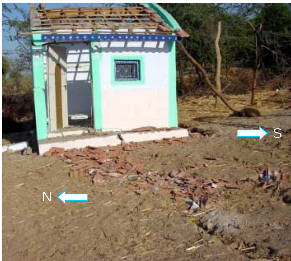
Figure 9. Extensional ground cracks crossing a small hut located in between the barren land and the corn field shown in Figure 8, with the corn field to the west.
