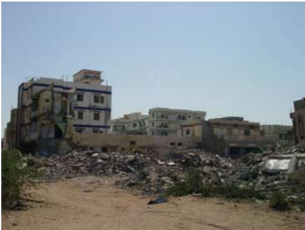
Figure 26. Buildings in different state of collapse and damage with wreckage dump in the foreground.
