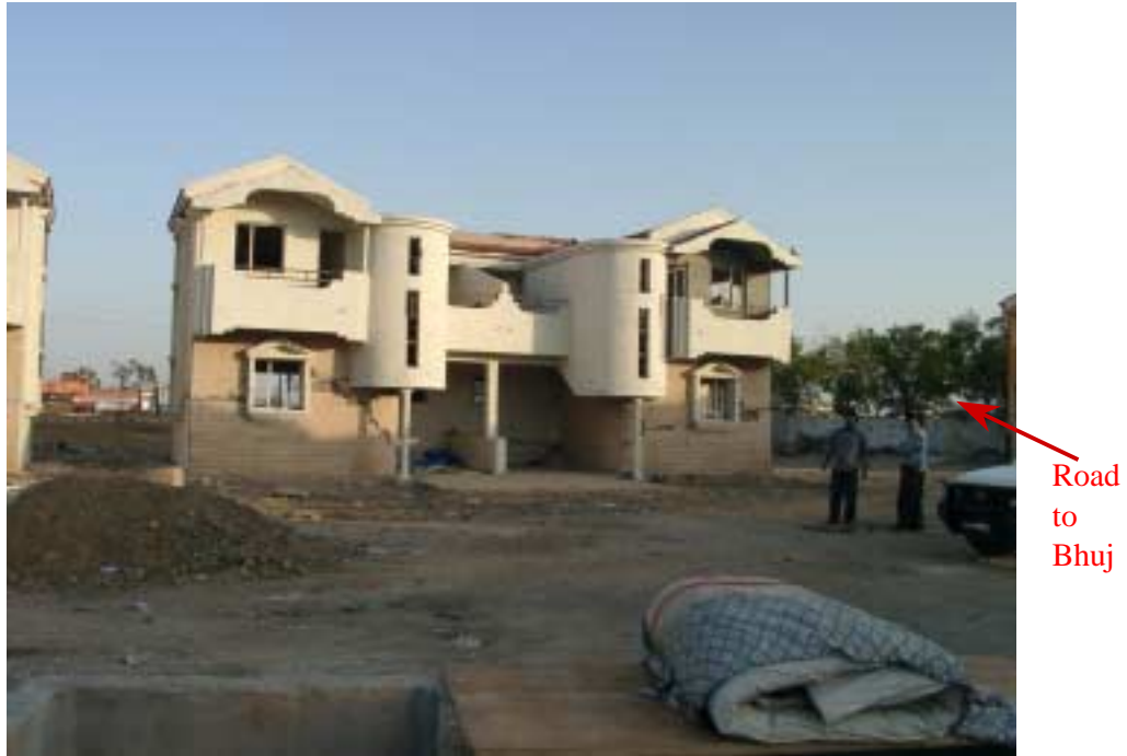
Figure 20. Severely damaged but still standing two housing unit block of the new housing complex shown in Figure 19. The small housing units are complete with parking lots, but the structural design does not seem to have considered seismic aspects. The bed seen outside is for the people guarding the property.
