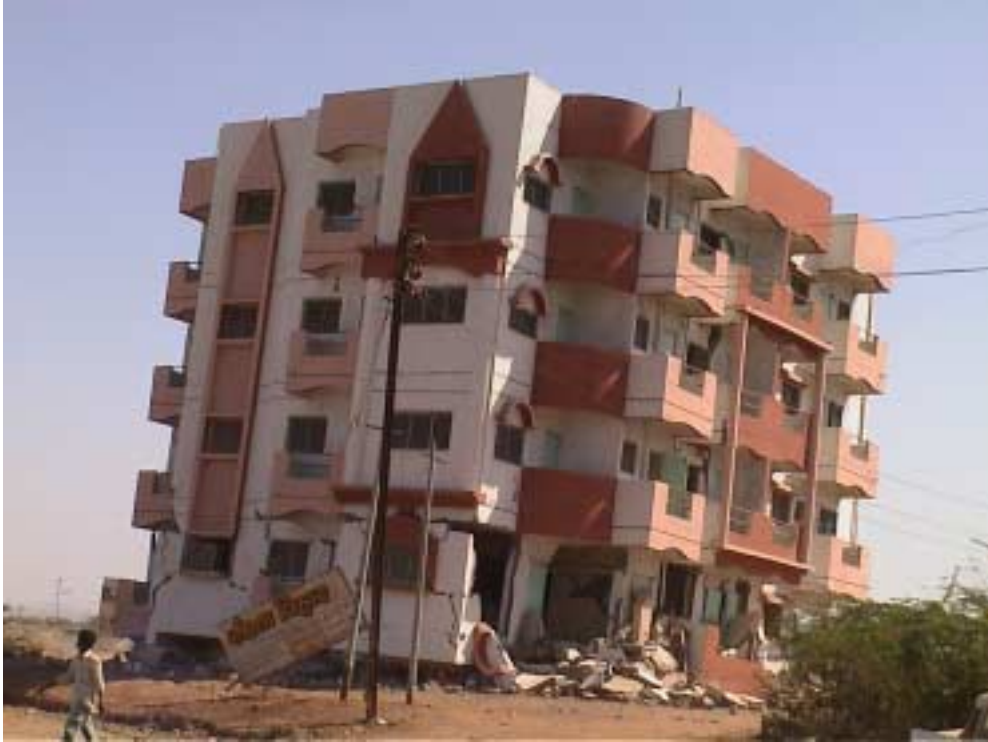
Figure 30. Apartment block consisting of reinforced concrete structure, severely tilted due to collapse of the first story. Apparently, the collapse resulted due to soft ground floor.
