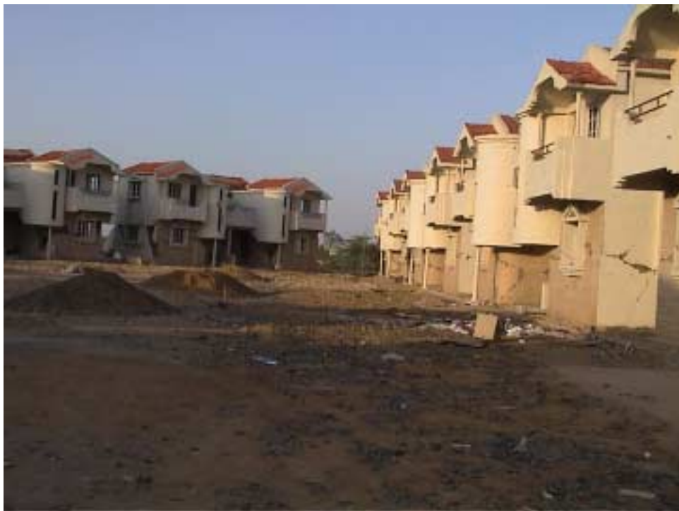
Figure 19. A new housing complex just ready for occupation, consisting of load bearing brick wall structures. The location is between Samakhial and Bhachau, about 80km east of Bhuj.
