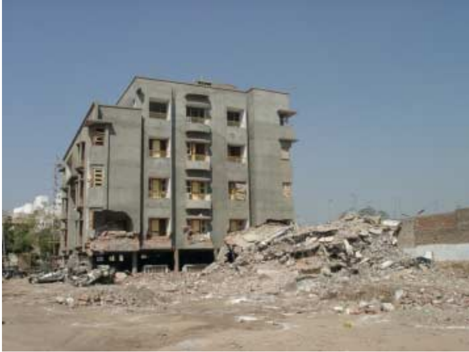
Figure 14. Wreckage of collapsed building and crushed vehicles parked in the open ground floor, near Maninagar station, south east of Ahmedabad. The adjacent building with open first floor parking space sustained some damage mostly due to the impact of collapsed building.
