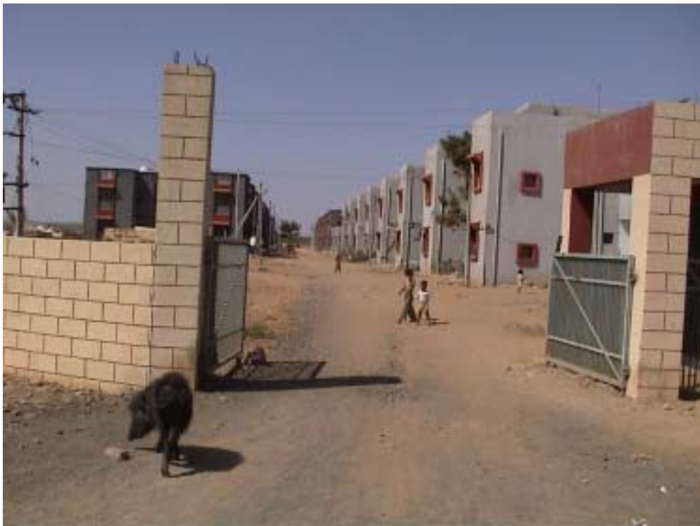
Figure 31. Housing complex with two-storied load bearing brick masonry structures in Bhuj, apparently still occupied after the earthquake.
