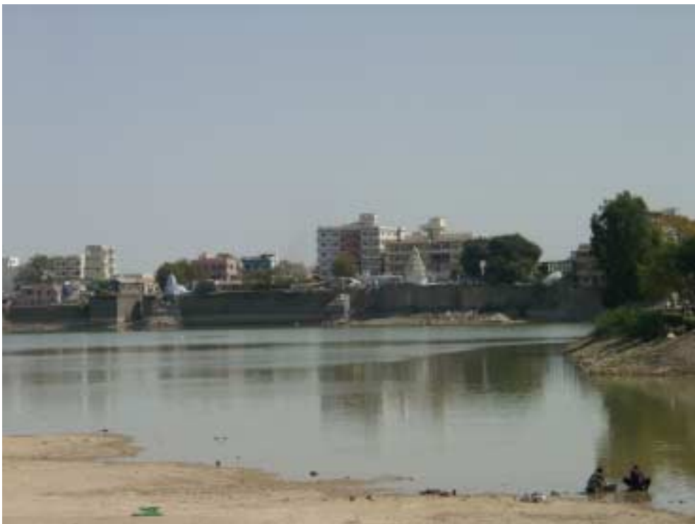
Figure 33. View from the lakeside in Bhuj facing south. Although it was not possible to inspect all the buildings closely, some of the structures in the background seemed to have resisted the earthquake shaking without large scale damage.
