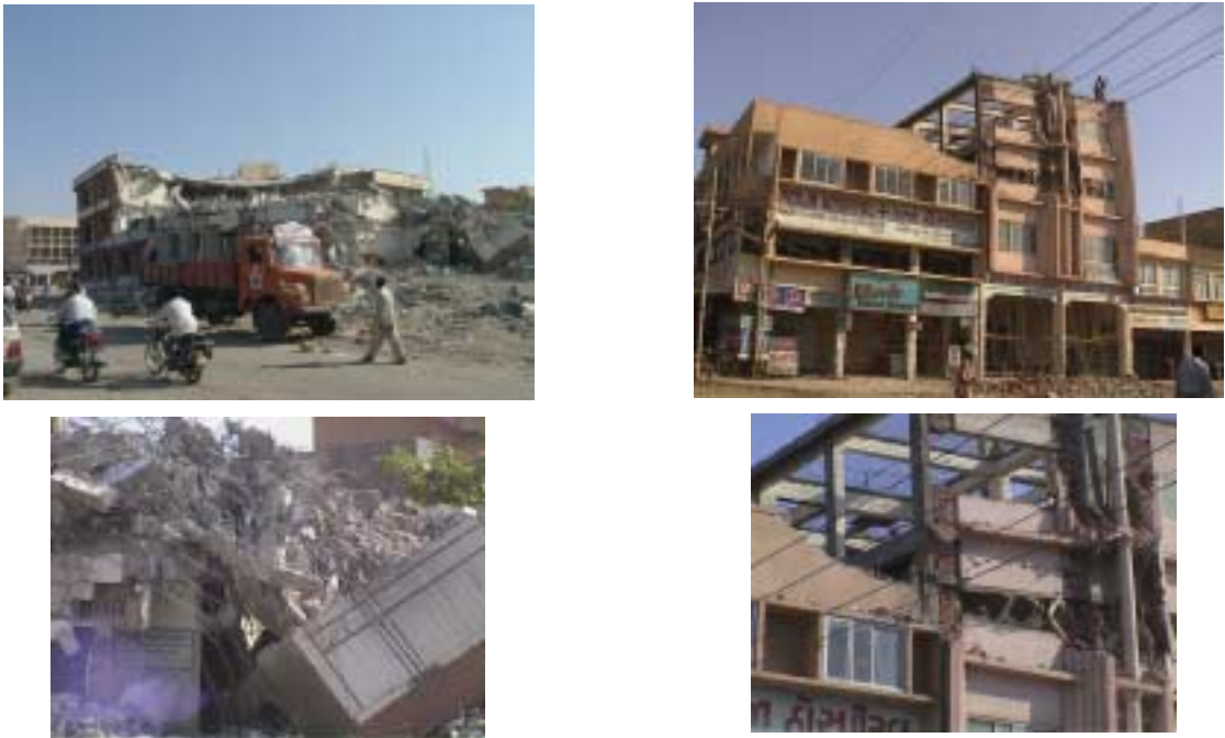
Figure 43. Demolition & removal of wreckage (left) and manual demolition in progress of a damaged hospital building with mid-floor collapse in Gandhidham. Clear separation of concrete & steel in the reinforced concrete wreckage (left) and demolition with hand-held hammer by the man standing at the top (right) provide some indication of the quality of materials used.
