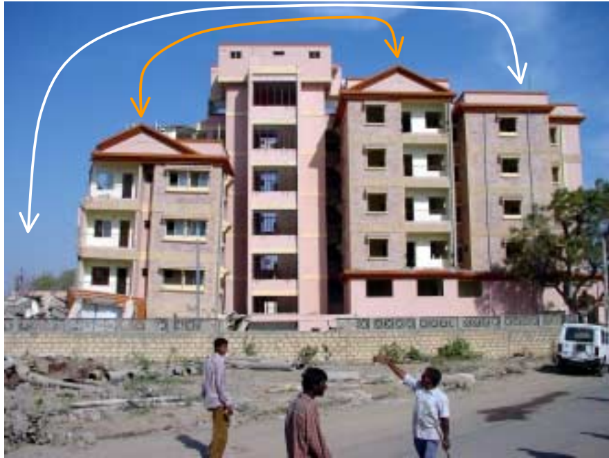
Figure 40. Partly collapsed and badly damaged new reinforced concrete building in Anjar just opposite (to the north) of the pigeon house shown in Figure 39. It seemed the building was designed to be more or less symmetrical on both sides of the stairs at the central part.
