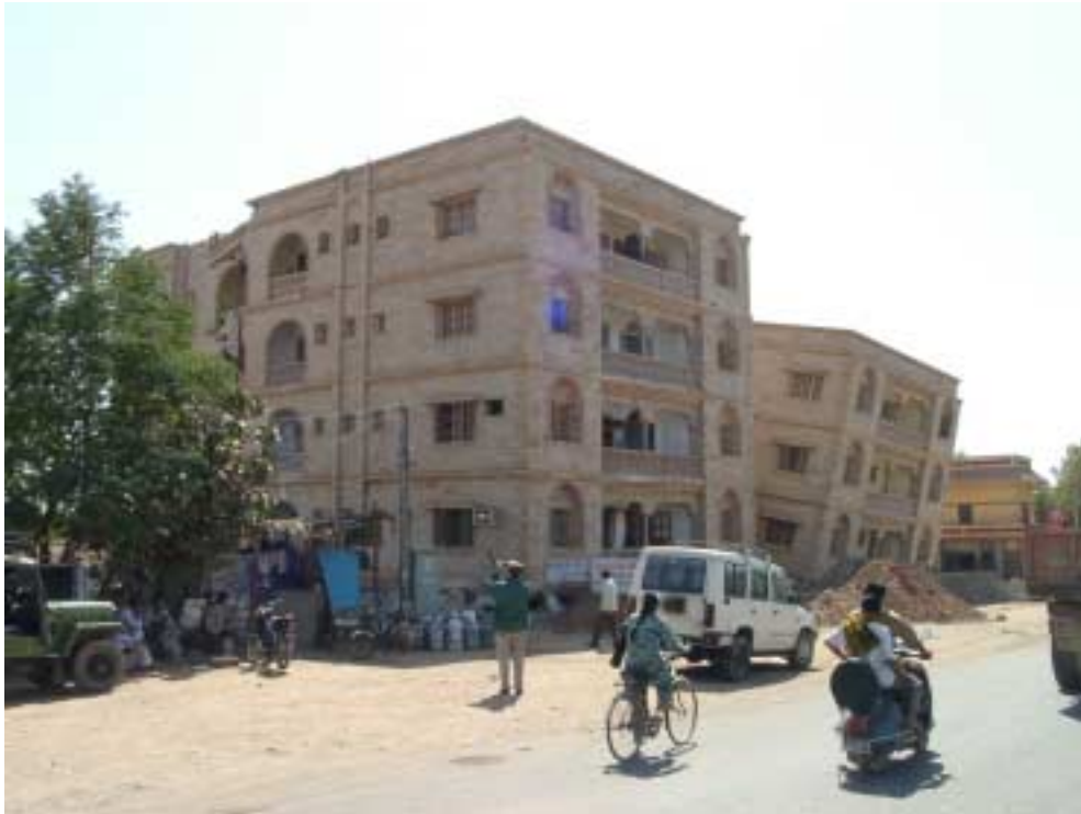
Figure 36. Overall view of the collapsed first story and tilting of relatively new concrete buildings with open space in the ground floor for shops and the like, creating a soft ground floor.
