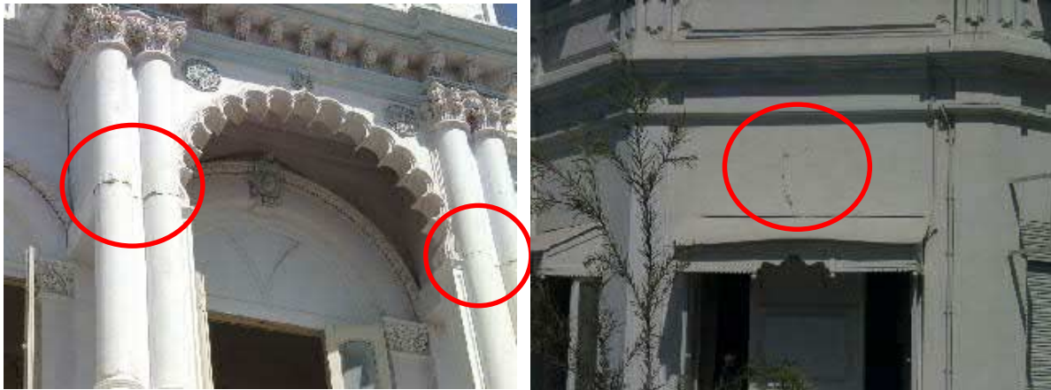
Figure 17. Closer look at the cracks on the exterior walls of Hotel Aram building. The cracks and damages on interior walls may have been more severe at sections the owner had already undertaken repairs and covered with cement mortar.
