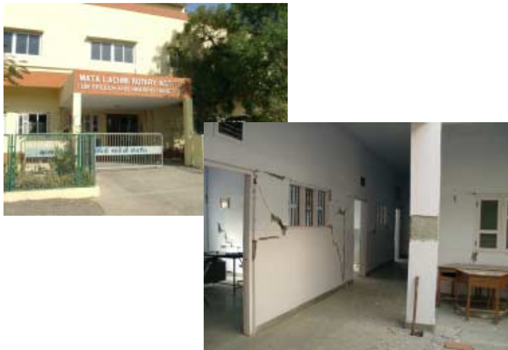
Figure 42. Frontage and the inside of Rotary institute for speech and hearing handicapped. The institute was closed after the earthquake, but the director who was kind enough to guide the authors the inside was planning repairs. Mostly, the damage seemed repairable.
