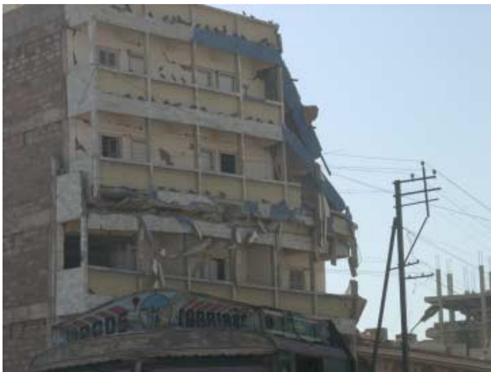
Figure 27. Partly collapsed massive concrete framed building structure with infill brick masonry walls.
