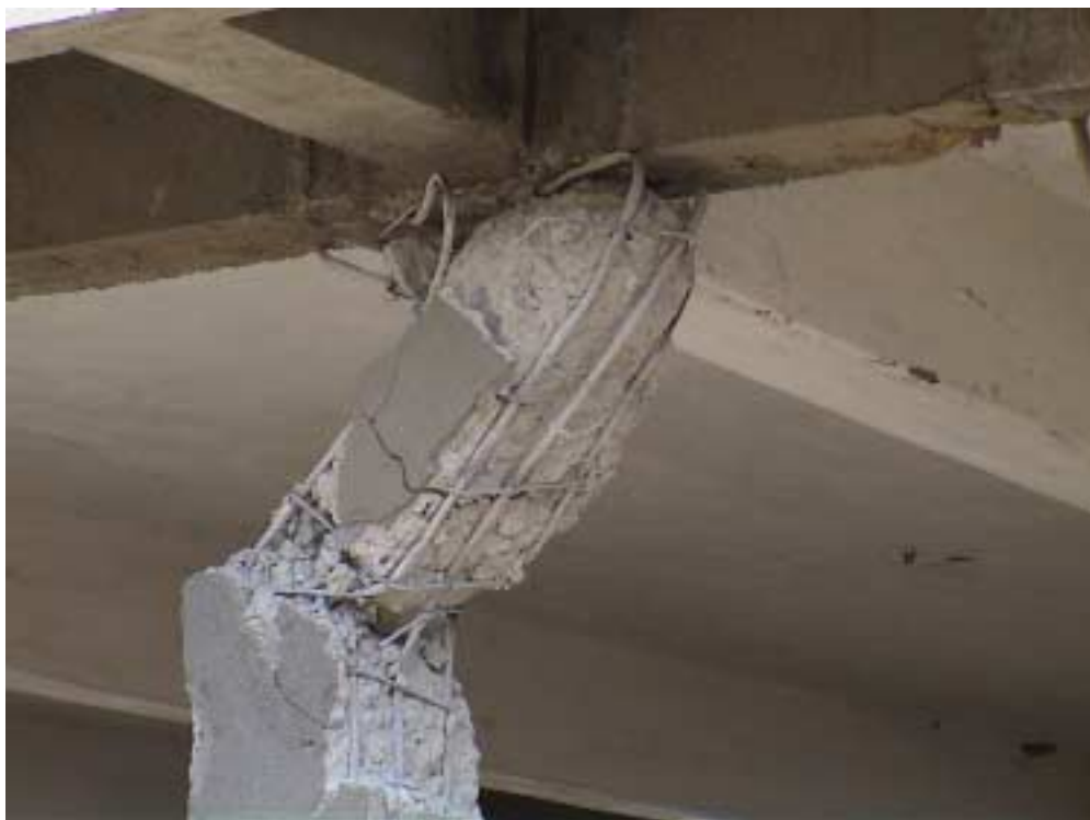
Figure 25. Close-up view of the top of concrete column supporting the factory building of Figure 24, showing the reinforcement details and concrete quality, and a substantial southward movement. The large southward movement may be due to stronger north south motion.
