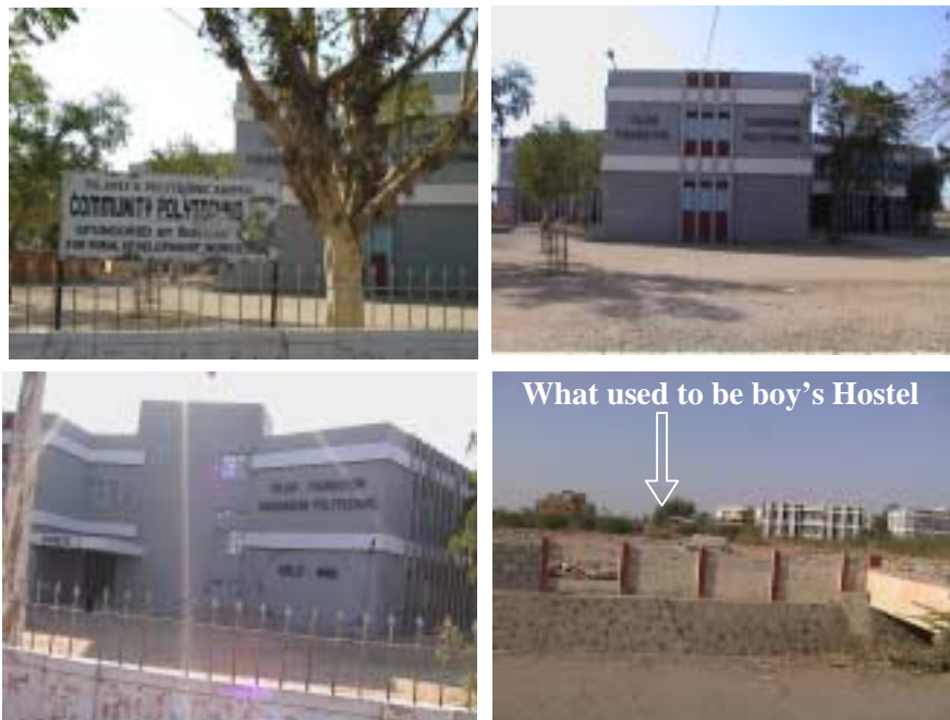
Figure 40. Damage and disruption at the polytechnic in Adipur where the girl's wing survived with severe cracking, but the collapse of boy's hostel resulted in a very large casualty.
