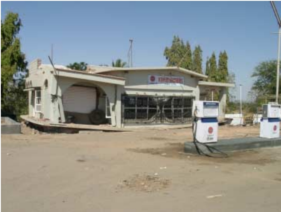
Figure 22. Collapsed office building of gasoline station near Bhachau. The gas station was in operation.
