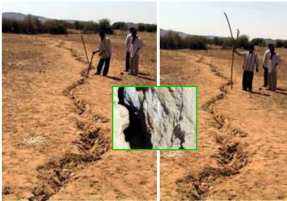
Figure 6. Extensional deformation over alluvial deposit observed near Lodhai. The inset shows the close-up view from within the cracks, where the evidence of salt-water expulsion may be noted from the salt deposit after evaporation.
