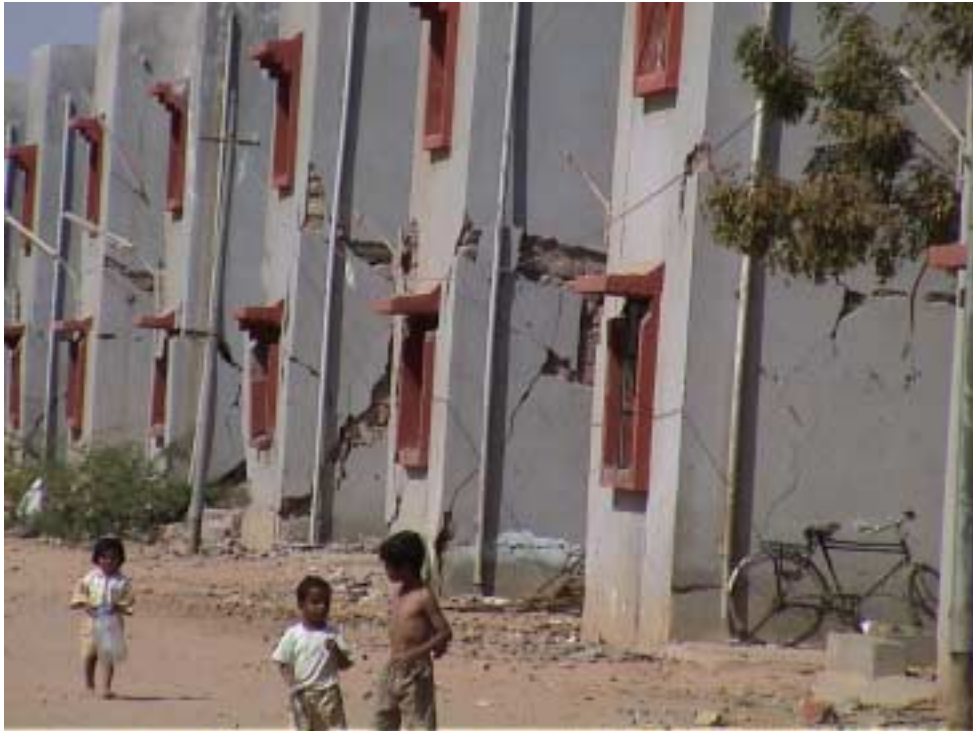
Figure 32. Closer view of the brick masonry housing units seen in Figure 31. Although severely cracked, the brick masonry housing units seem to have been kept from complete collapse.
