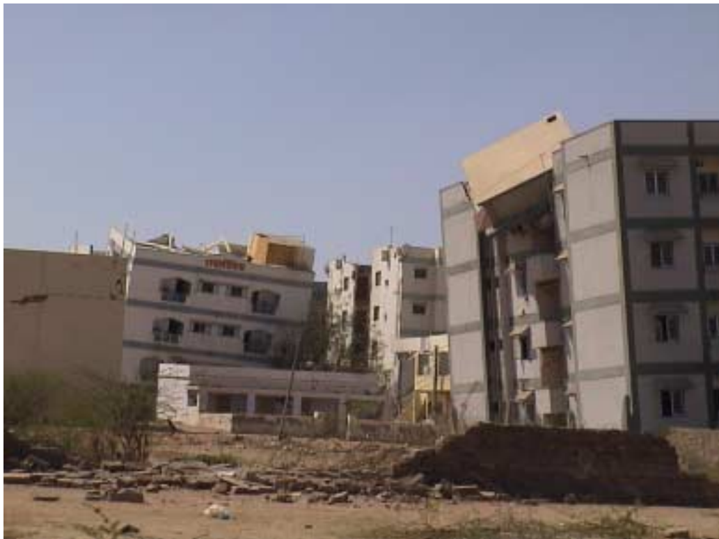
Figure 29. Close-up view of Figure 28 showing tilted buildings and toppled overhead water tank.
