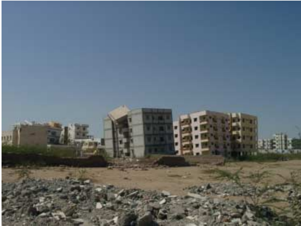
Figure 28. Group of damaged, tilted & partly toppled apparently relatively new apartment blocks in the central part of Bhuj. Damages to some of the buildings in the group seemed to be repairable.
