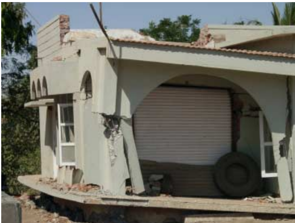
Figure 23. Closer view of the collapsed building of the gasoline station near Bhachau.
