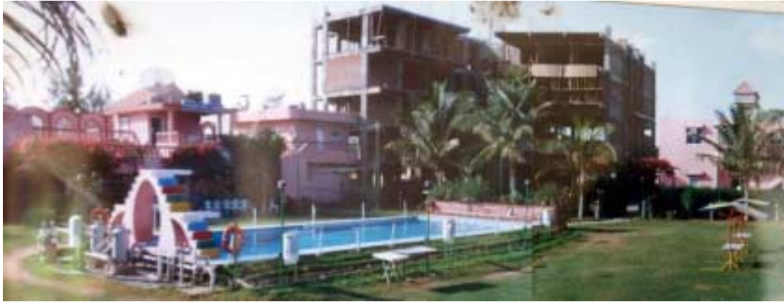
Figure 47. View of the collapsed block at Sharma Resort during construction. Again a photograph from the picture the owner kindly showed the authors. It is clear that the building consisted of reinforced concrete frame structure with infill brick masonry wall. This system of construction is typical of the reinforced concrete buildings in the region.
