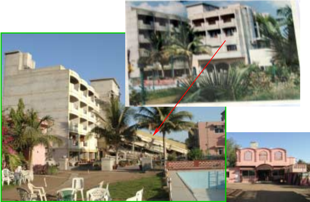
Figure 45. The collapsed wing of the luxury resort that was still in business, where authors spent overnight. The top inset is a photograph taken from the photograph the owner was kind enough to show to the authors and shows how the building looked before collapse. The inset to the right is the entrance to the reception area.
