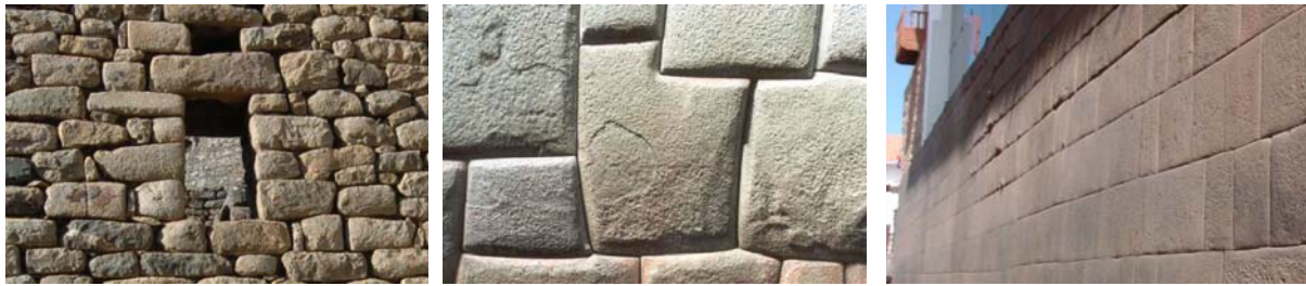
(a) Roughly shaped stone masonry
