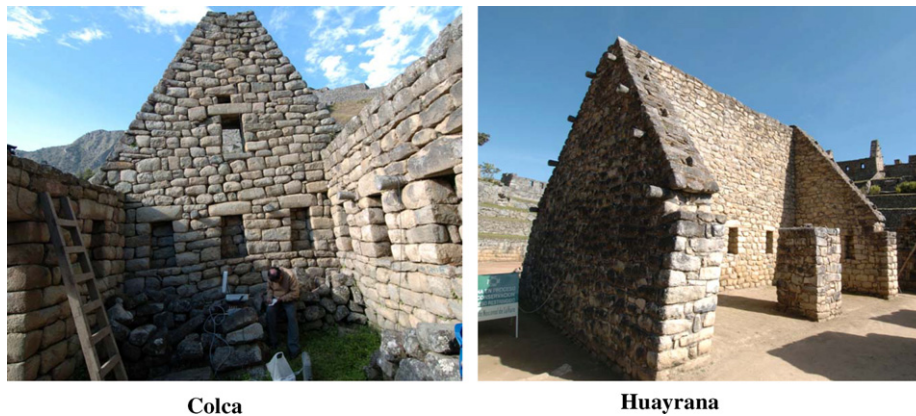
Fig. 11. Selected buildings for analysis of Inca's stone structures.
