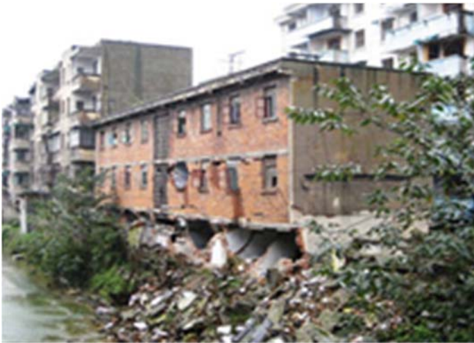
A brick wall collapsed during an earthquake. These photographs of collapsed brick walls in Sichuan Province, China, were taken immediately after a M7.9 earthquake occurred at 14:28, May 12, 2008.
