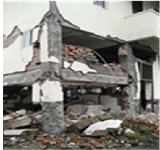
A brick wall collapsed during an earthquake. These photographs of collapsed brick walls in Sichuan Province, China, were taken immediately after a M7.9 earthquake occurred at 14:28, May 12, 2008.
