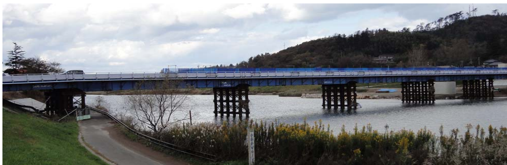
Experiment point of bridge
